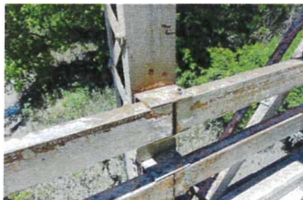
Conditions of existing bridge
